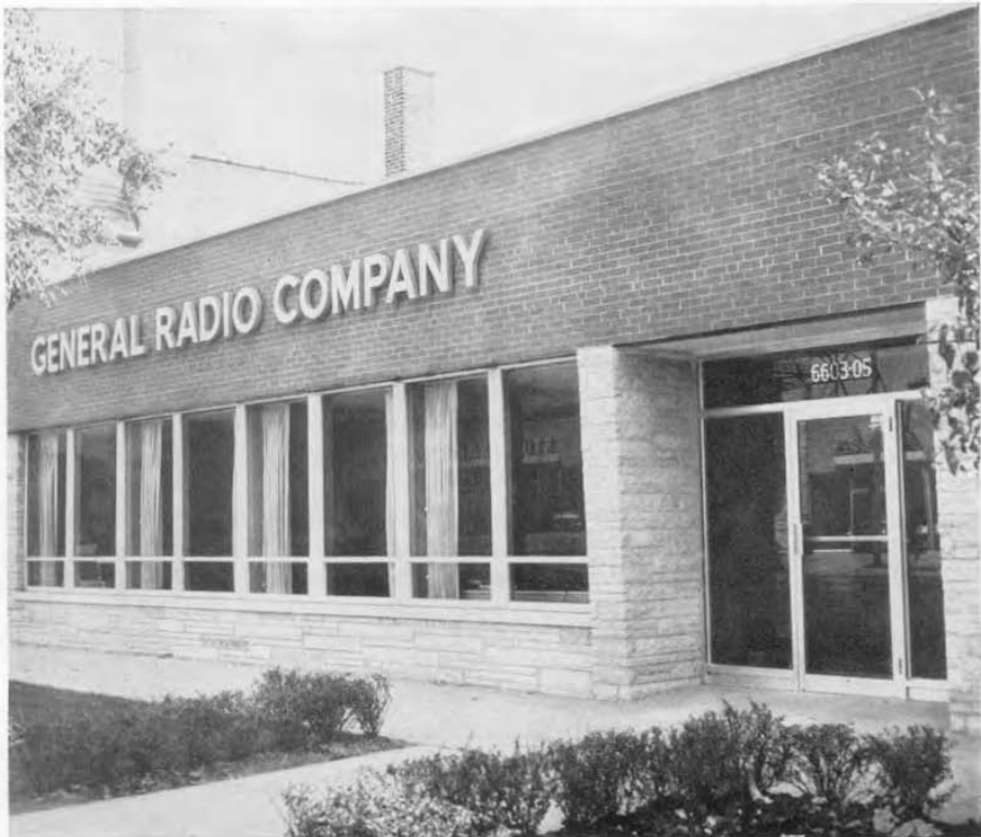
View of the new front door — 6605 West North Avenue, Oak Park, Illinois.
